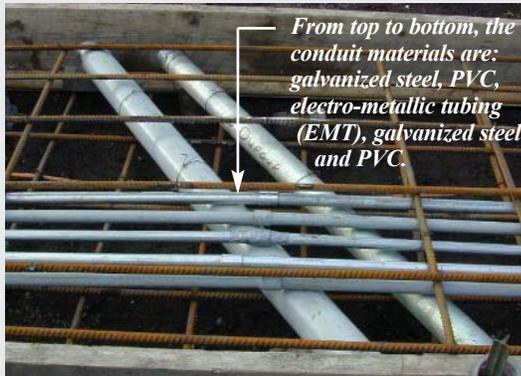
**Figure 1:** Test site prior to concrete pouring. There are five conduits running from left to right, all 1" diameter.
