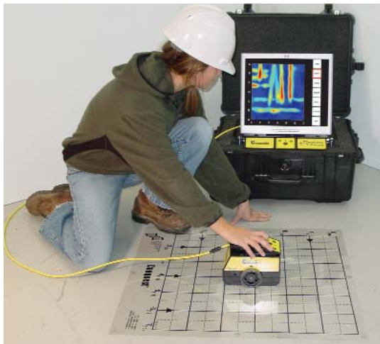
Figure 2: Scanning a Conquest™ grid on the site after the concrete pour.
