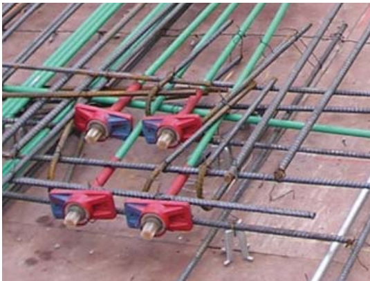
Figure 1: Site construction prior to concrete pour.
